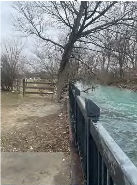
PHOTO NO. 8: Looking N from SE corner of 14702 Riverside Boulevard
