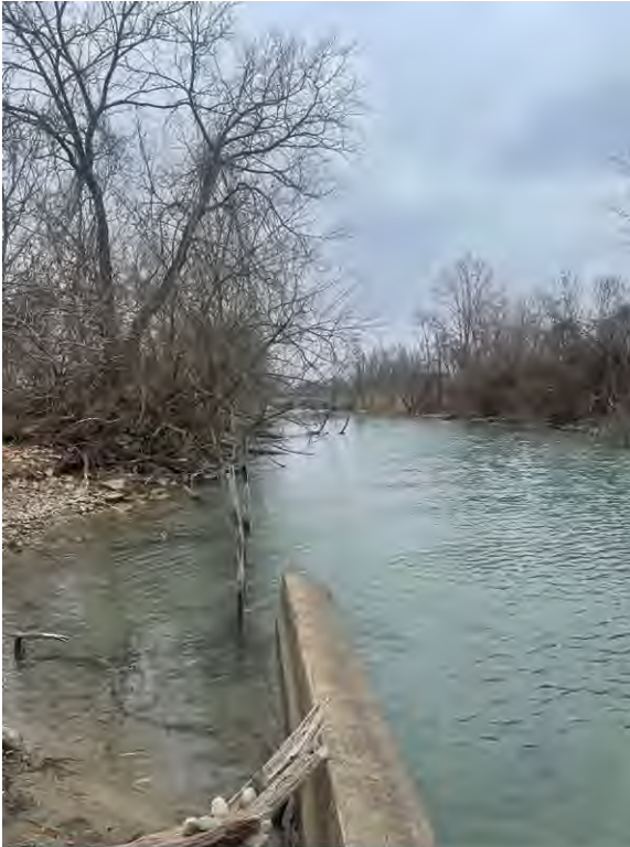
PHOTO 15: Looking N from N end seawall at 100 Lenox
