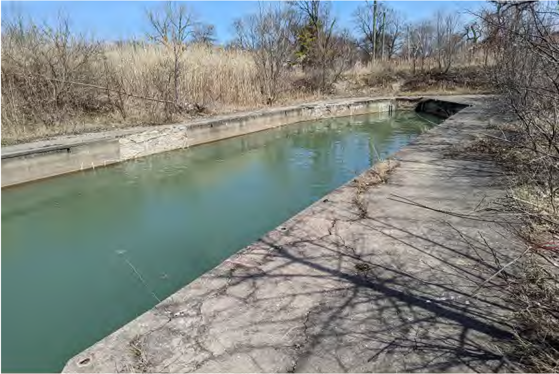
PHOTO NO. 7: North Bay
