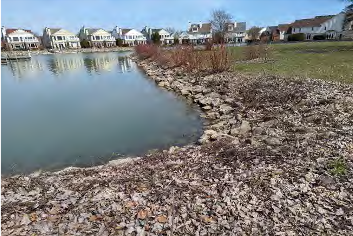
PHOTO NO. 3: More Riprap
