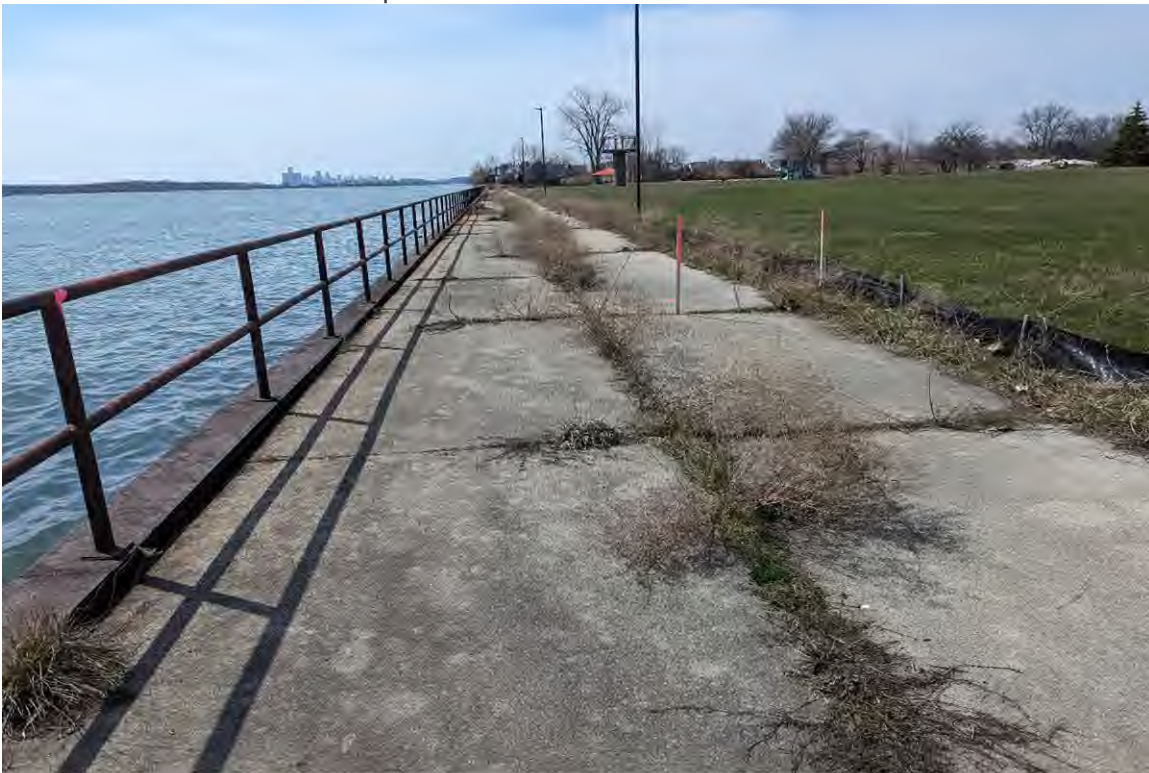
PHOTO NO. 10: General picture looking west.
