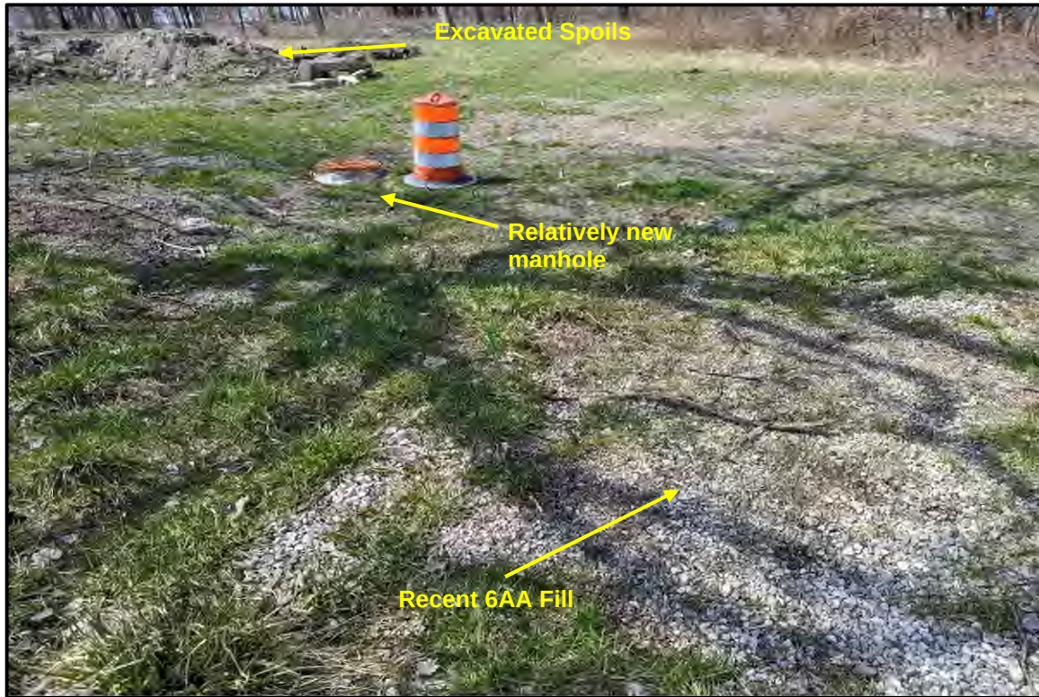
PHOTO NO. 1: Recent Sewer Repair
