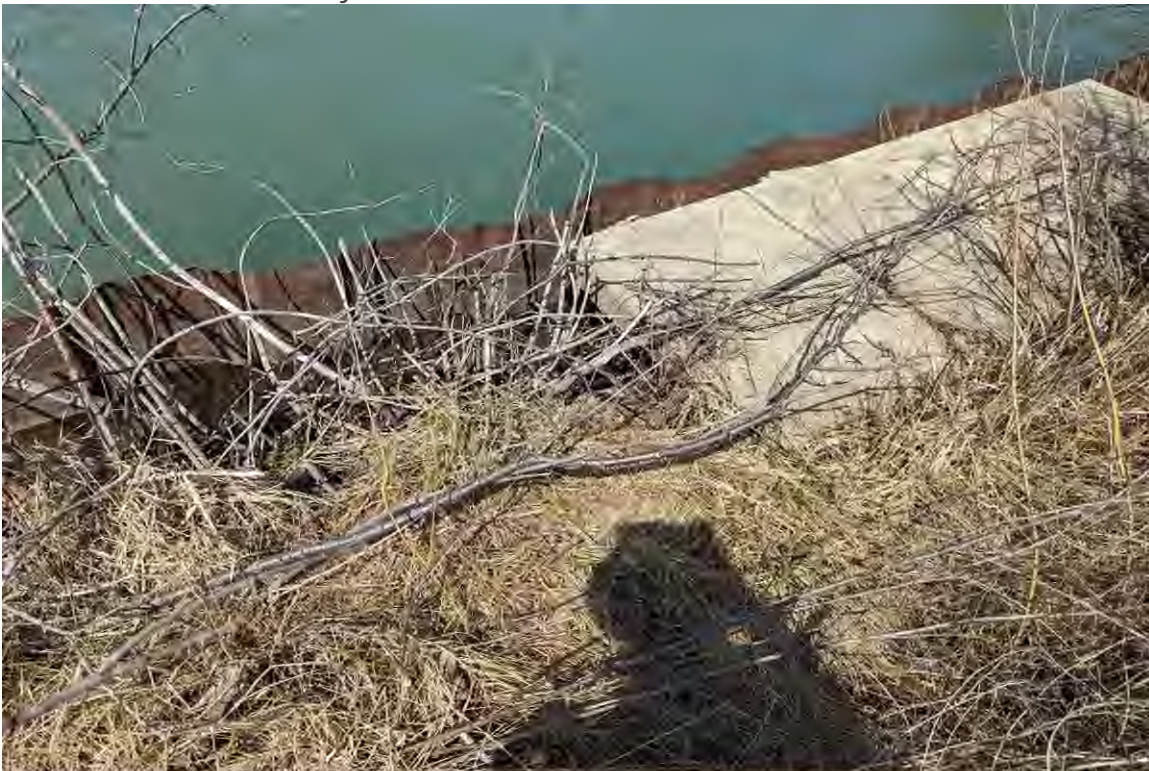
PHOTO NO. 10: Steel sheeting along channel and into north bay
