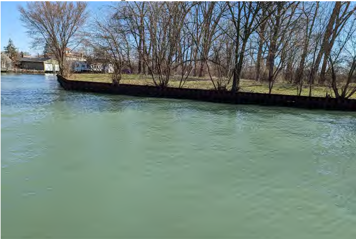
PHOTO NO. 2: Seawall of opposite side of channel
