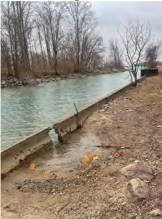
PHOTO 16: Looking S at seawall near midpoint of wall at 100 Lenox
