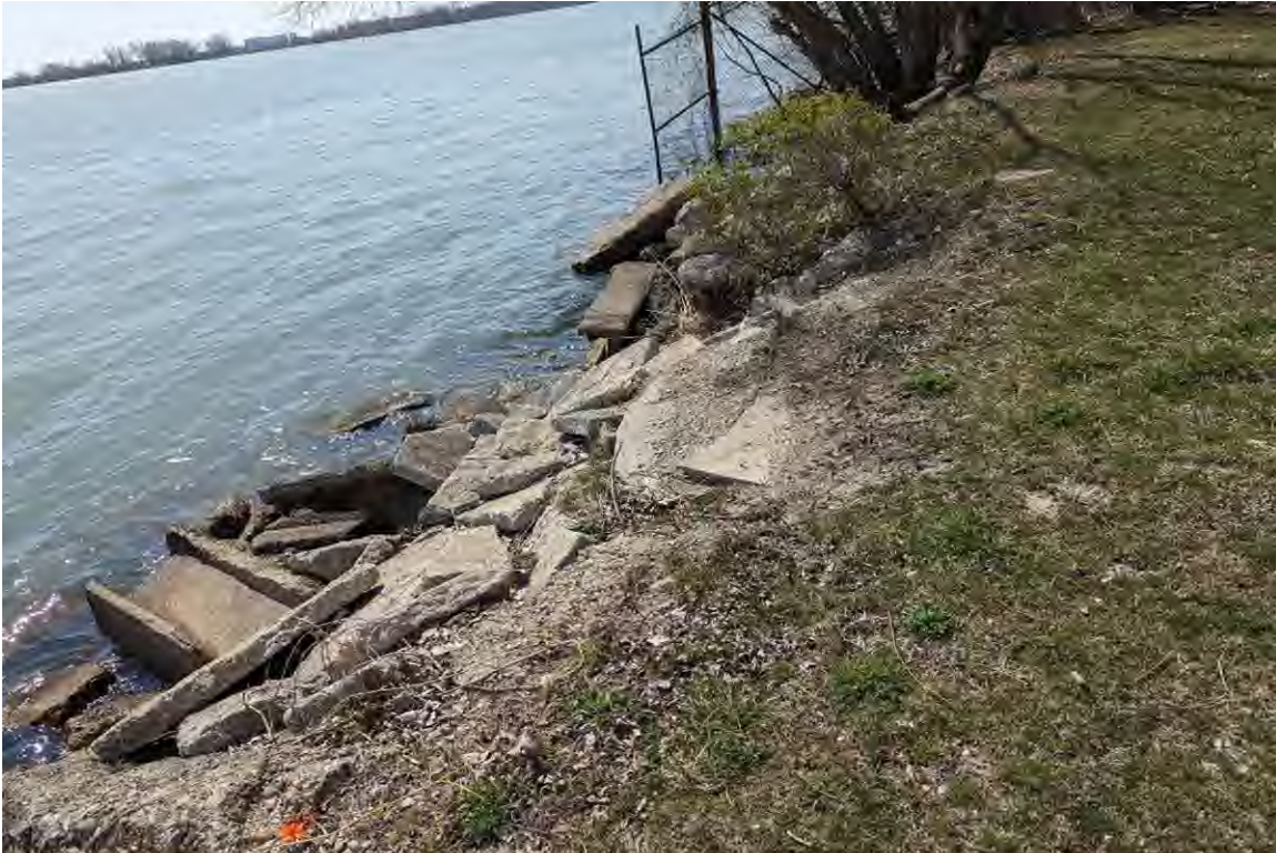
PHOTO NO. 1: No seawall. Concrete Riprap
