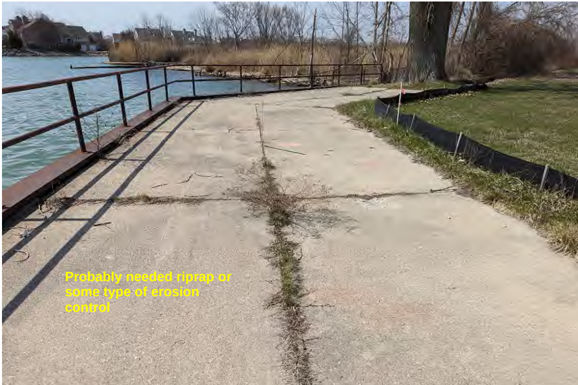
PHOTO NO. 3: General picture looking west.
