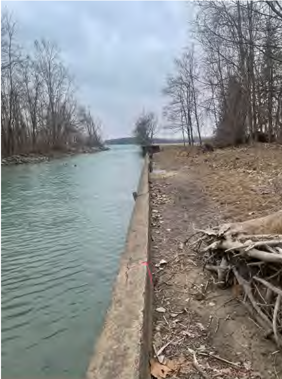
PHOTO 13: Looking S from center E side of 100 Lenox
