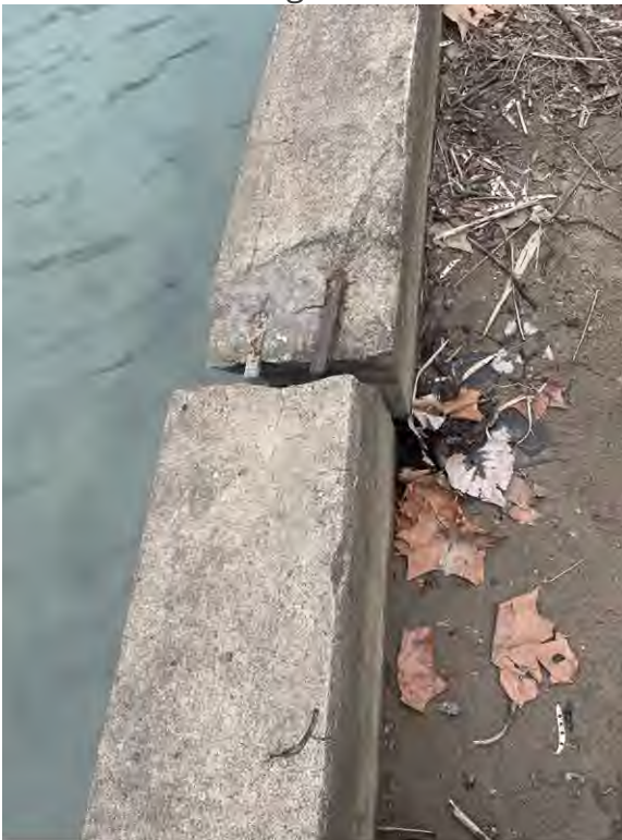
PHOTO 14: "Intact" concrete wall at S end 100 Lenox
