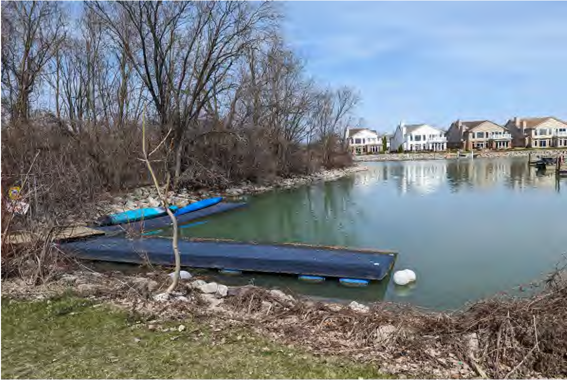
PHOTO NO. 5: Riprap along property boundary.
