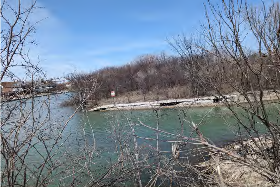
PHOTO NO. 9: North bay inlet
