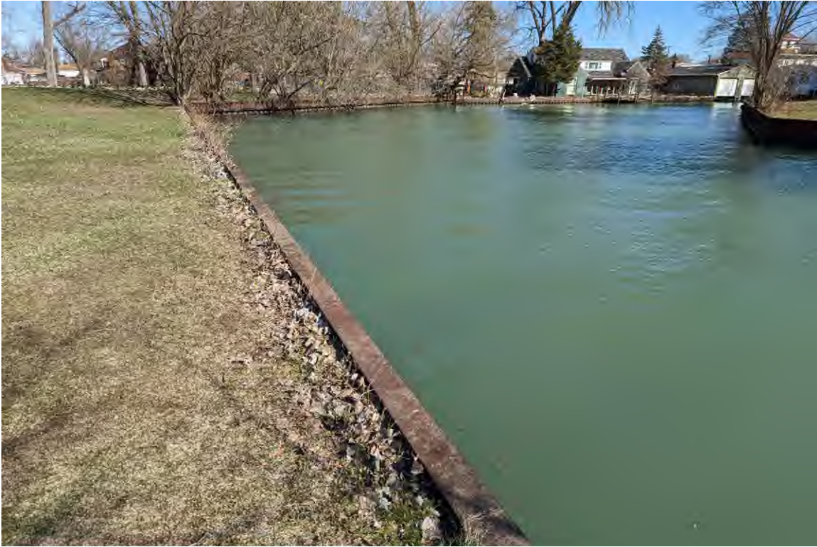
PHOTO NO. 1: Seawall along channel
