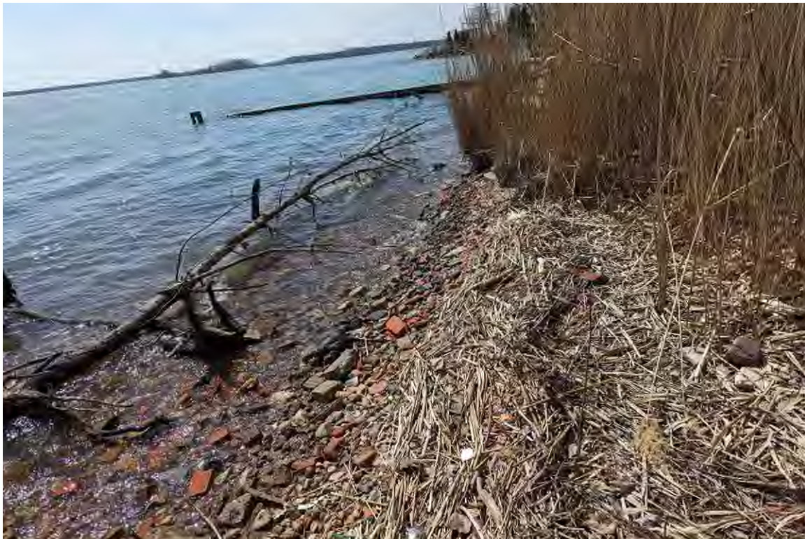
PHOTO NO. 22: Concrete Seawall extending to submerged section
