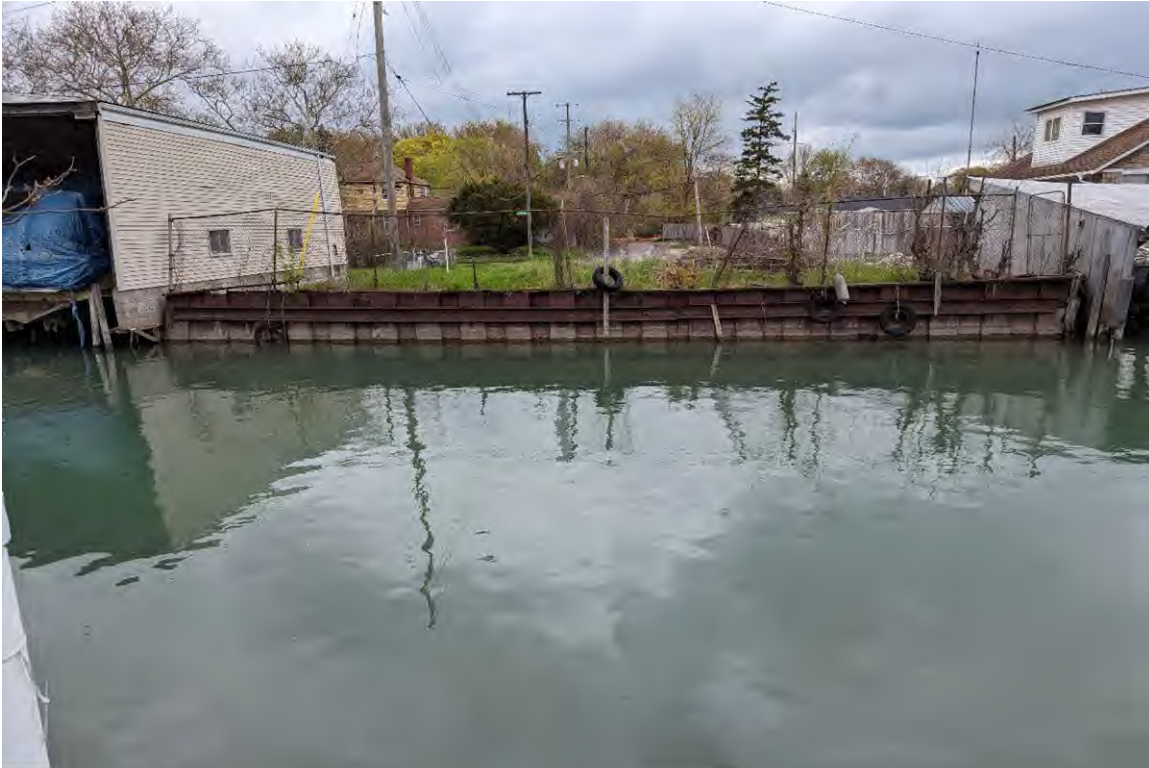
PHOTO NO. 3: Harbor Island Center Seawall from West Harbor Island.
