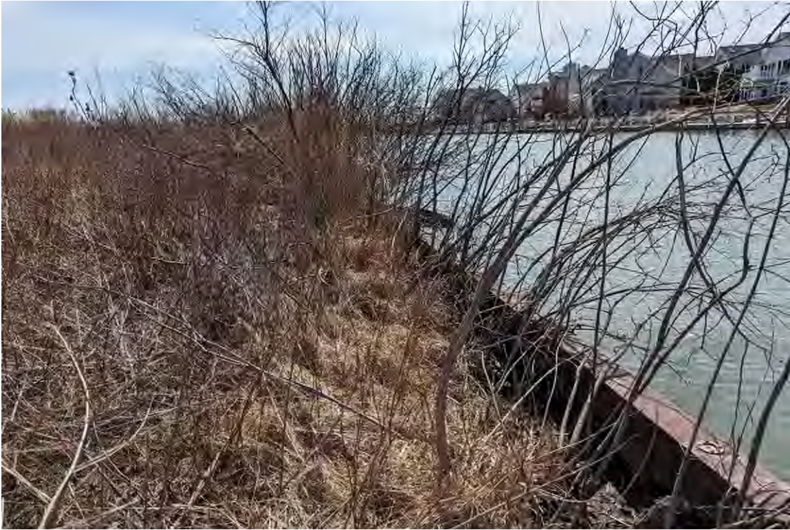
PHOTO NO. 11: Steel sheeting along channel
