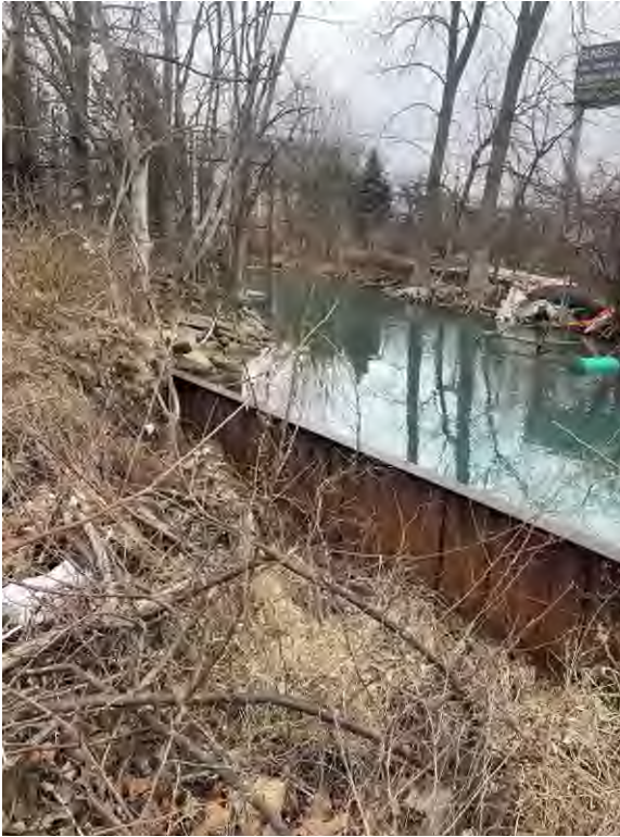
PHOTO NO. 1: Looking NE from 950 Manistique at 14728 East Jefferson
