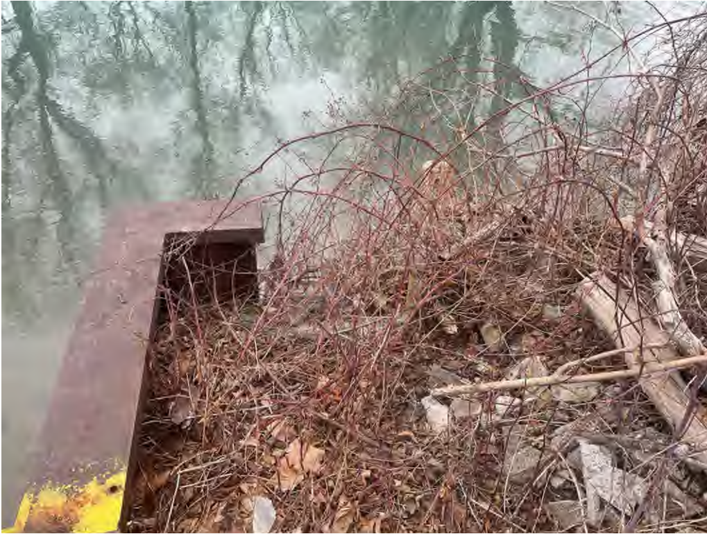
PHOTO 17: Wall at W End Klenk Island
