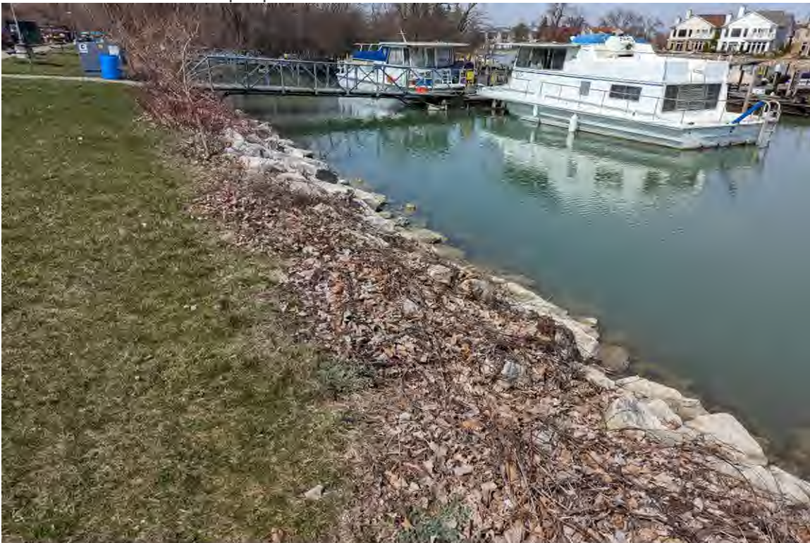
PHOTO NO. 4: Riprap by docks
