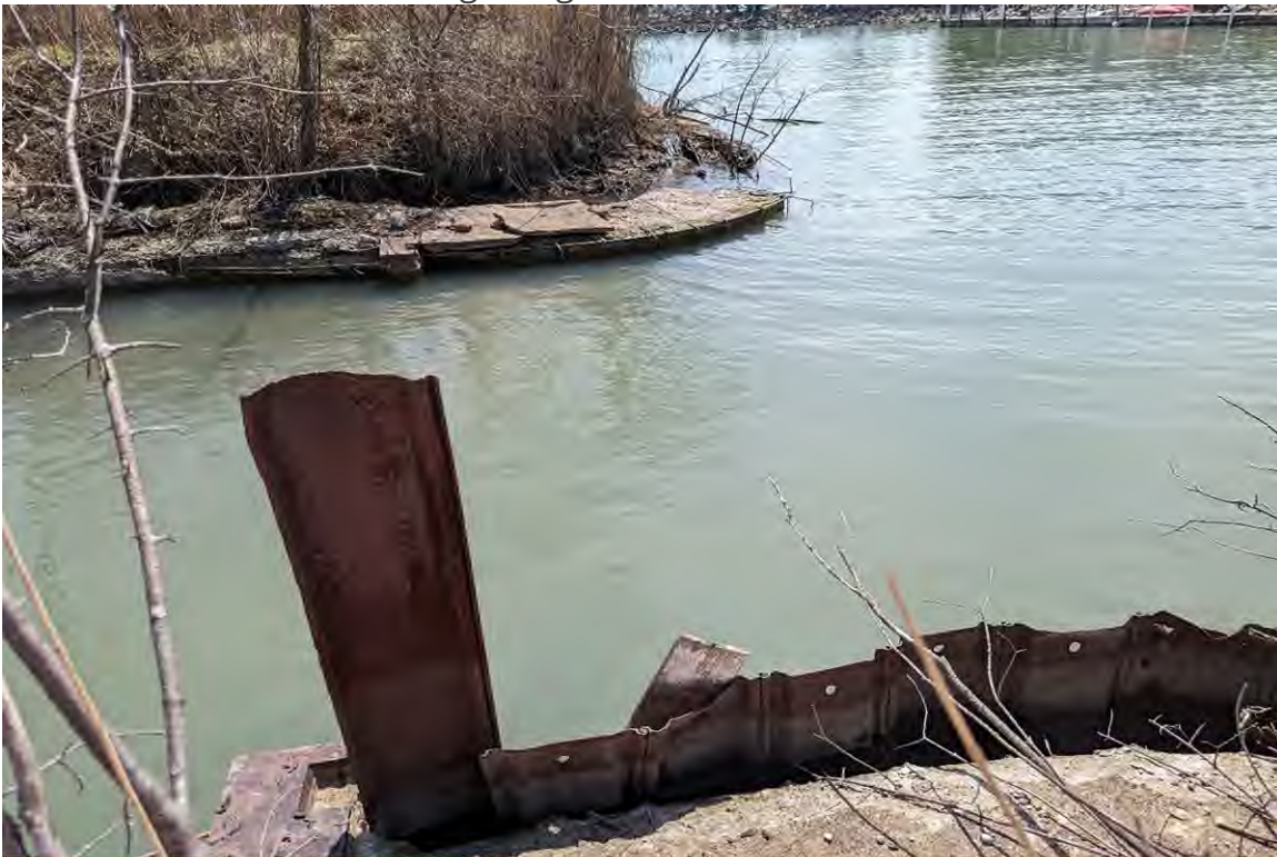
PHOTO NO. 12: Steel Sheetting into Middle Bay
