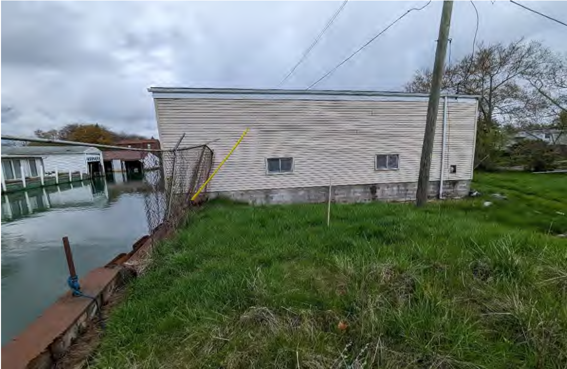
PHOTO NO. 5: Harbor Island Center north covered dock.
