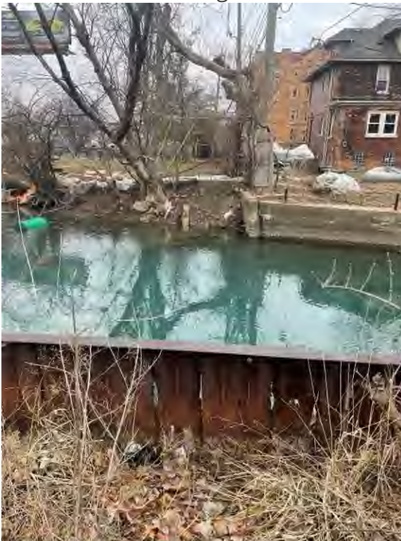
PHOTO- NO. 2: Looking E at south end of 14728 Jefferson from 950 Manistique
