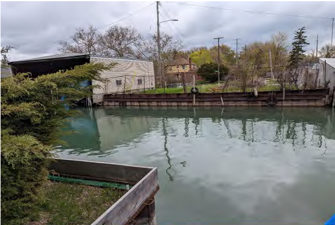
PHOTO NO. 4: Harbor Island Center Seawall from West Harbor Island.
