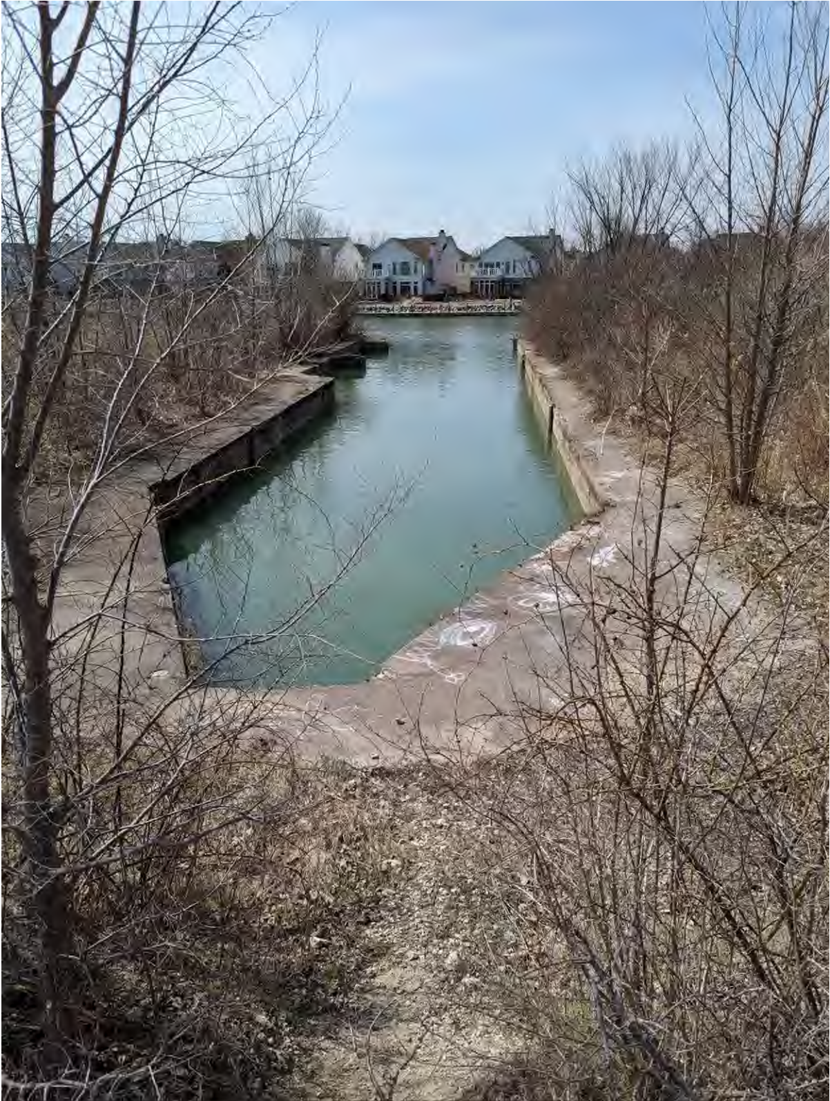
PHOTO NO. 6: North Bay
