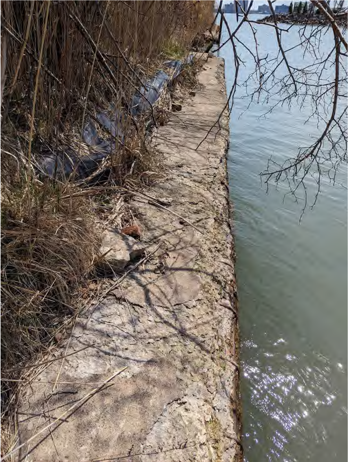
PHOTO NO. 15: Concrete Seawall along Channel
