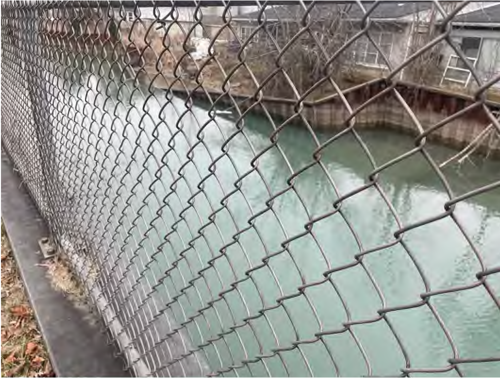
PHOTO NO. 7: Looking SW at 14818 Harbor Island Street.
