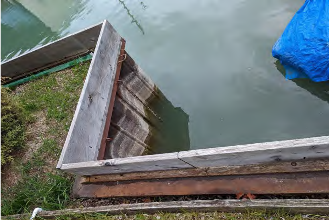
PHOTO NO. 1: West Harbor Island Center seawall from above.
