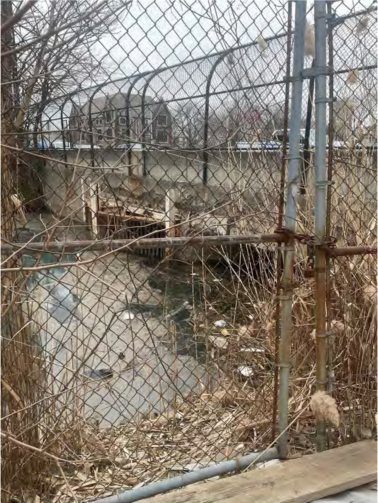
PHOTO 19: Looking W at N end 14728 East Jefferson Avenue
